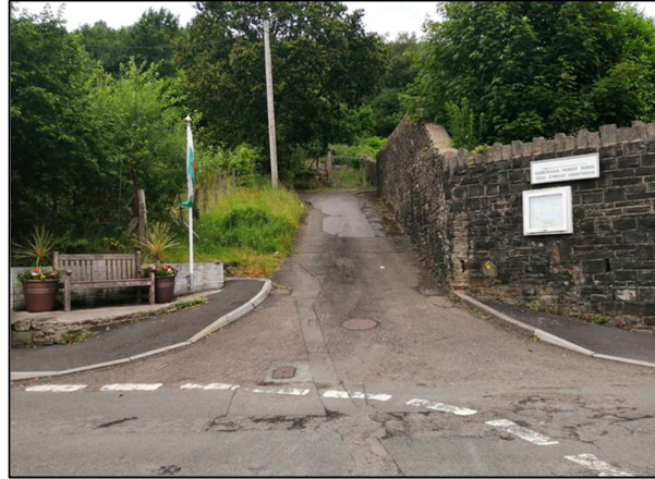
Insert 7: Existing School Entrance to be widened.
